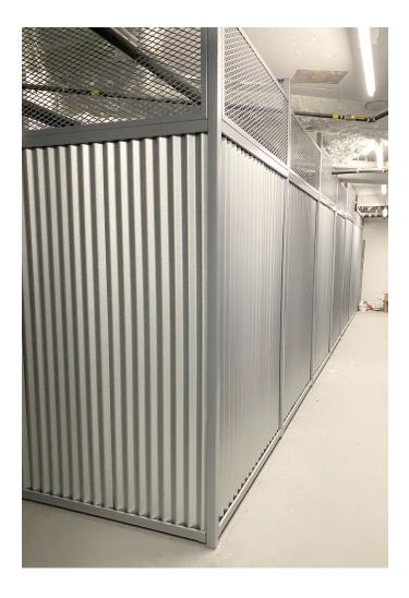
**Security Locker** walls are constructed from corrugated sheeting enclosed above and below by 2"sq steel channel. Coated in a durable Galvalume finish, the walls resist dirt, scratching and rust.
