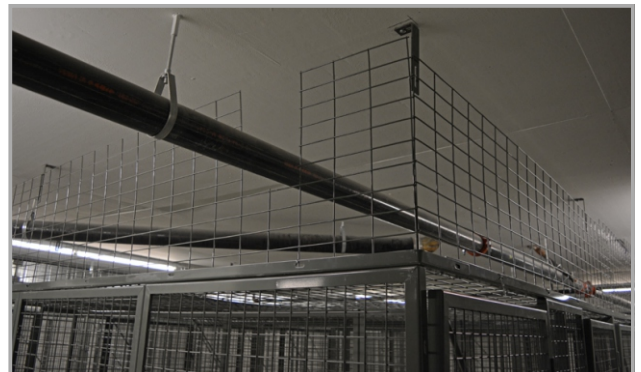
Wire Mesh Transom above lockers..
